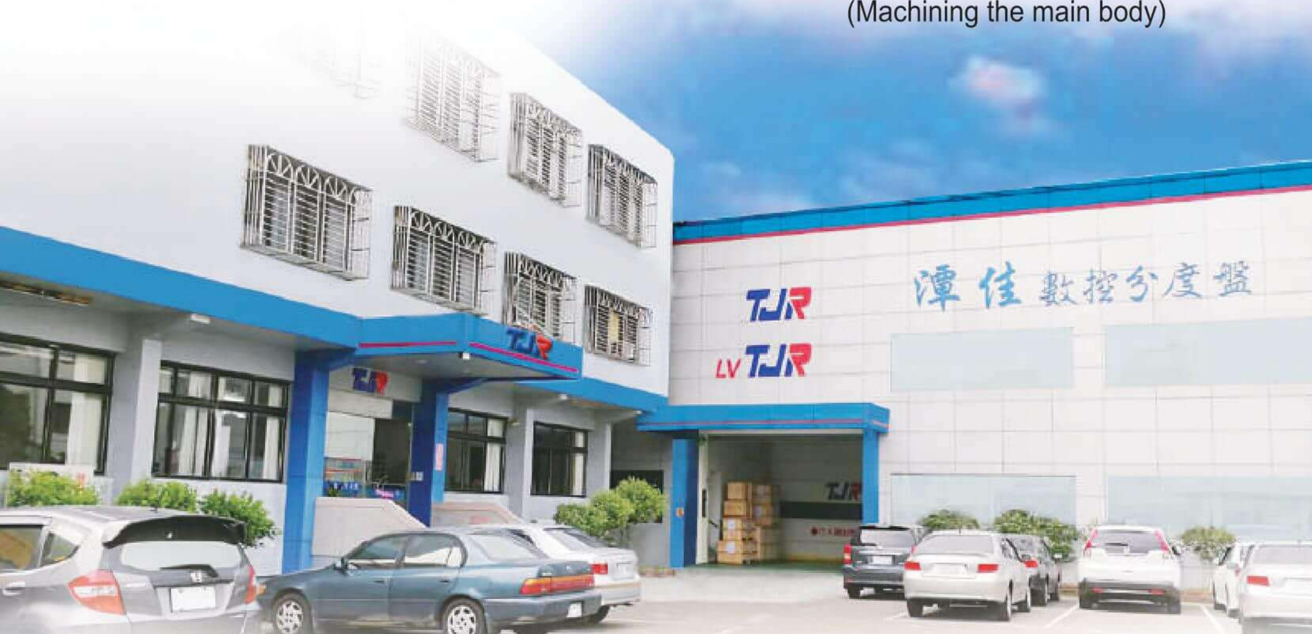
▲ Appearance of Taiwan Plant
